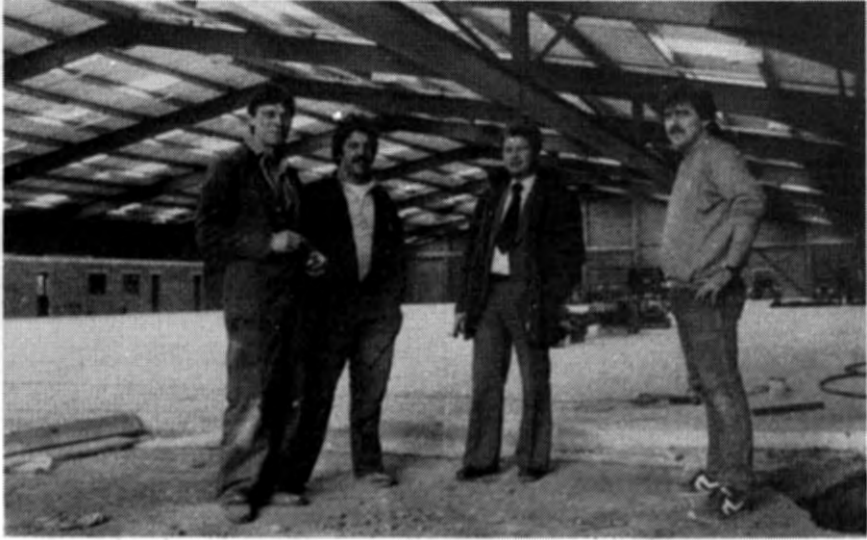
Pictured at the Southern Evans building, left to right, electricians Norman Dennett and David Gravener with engineer Lew Carter and Phillip Burquest, also an electrician.
